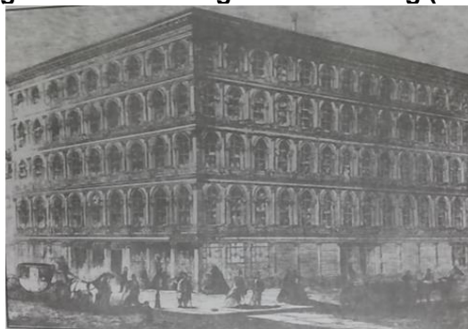
Figura 1 - E. V. Haughwout Building (1857)
